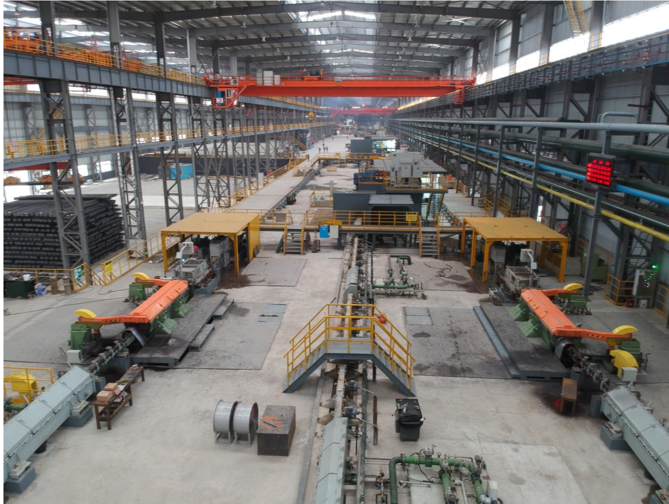
High Speed Rebar Mill with 4-stand 250 eDrive NTM
